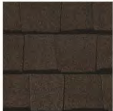
ASPHALT SHINGLE ROOFING
